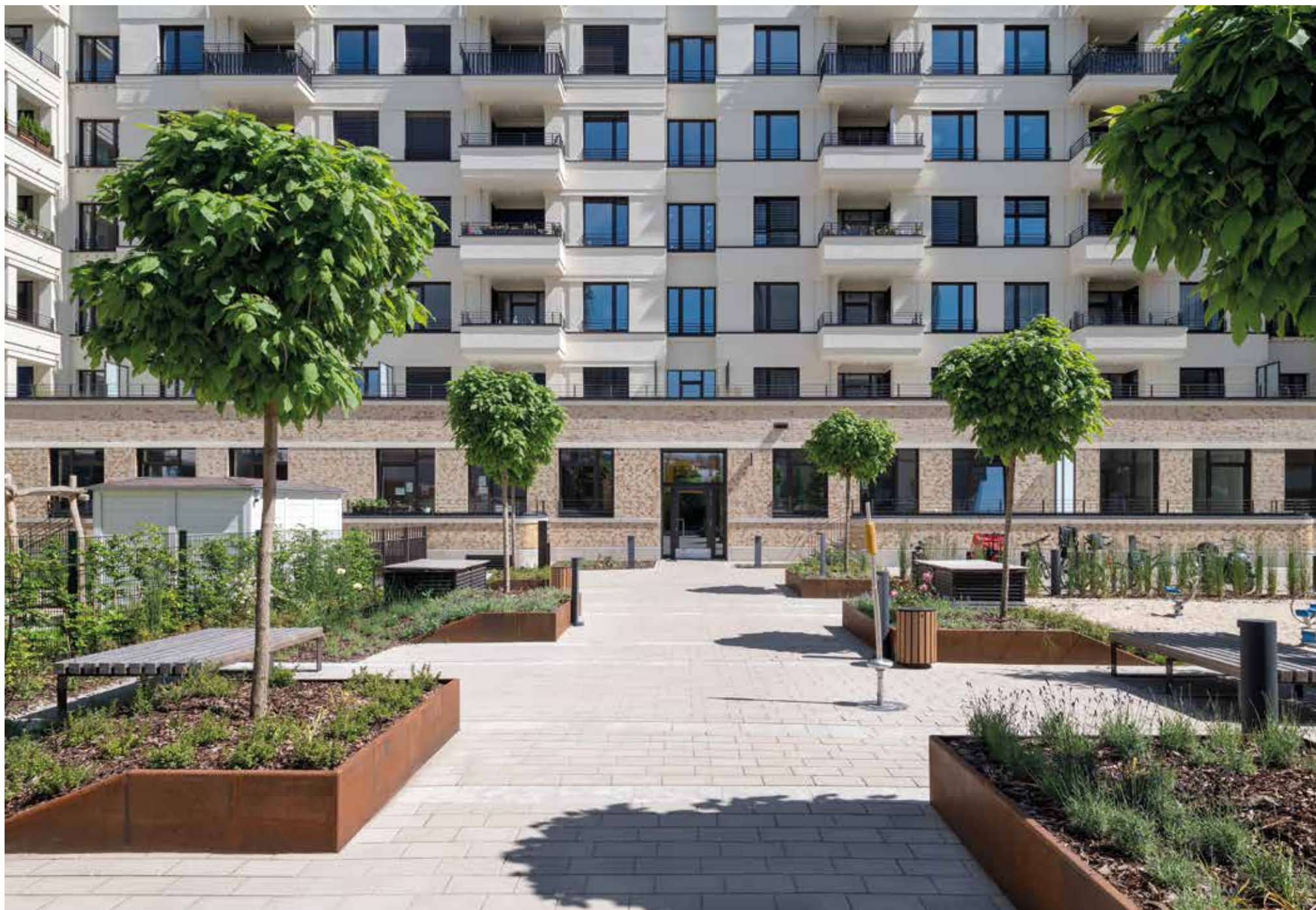
GDM. SCADA aBG Nr. Z-84.1-29 proActive 30/20/8 a 20/20/8 cm s 8mm spárou, silco, vápenec, proWater, proDrain
